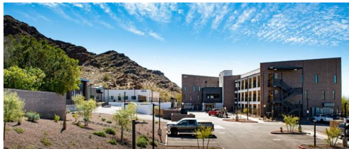
Patina Mountain Reserve in Phoenix, Arizona, is the new construction of a 48-bed community situated on the edge of the Phoenix Mountain Preserve area. Residents have access to integrated medical care and support services focused on the Native American community.
