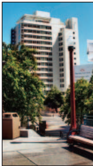
View of the new International Hotel from Portsmouth Square in San Francisco's Chinatown.
